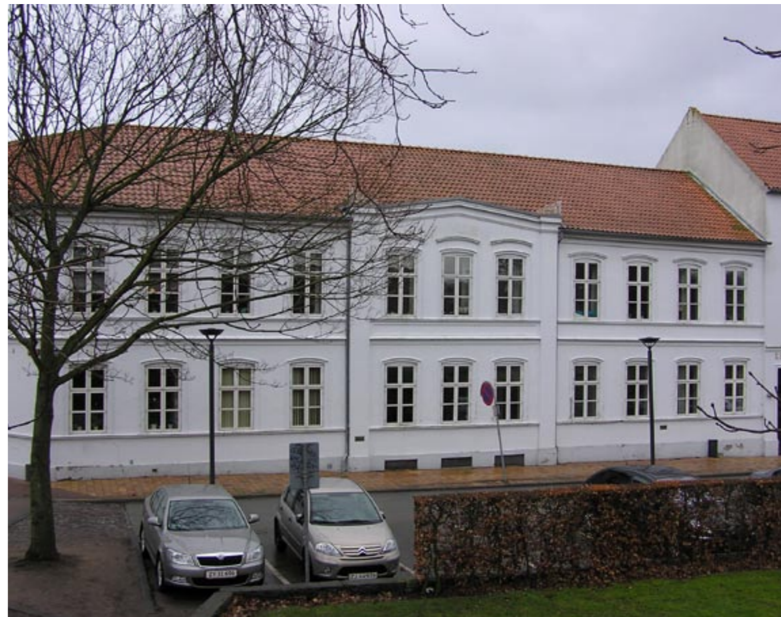
Vestfacade mod gade
